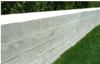
⑥ CONCRETE RETAINING WALL, HEIGHT VARIES
